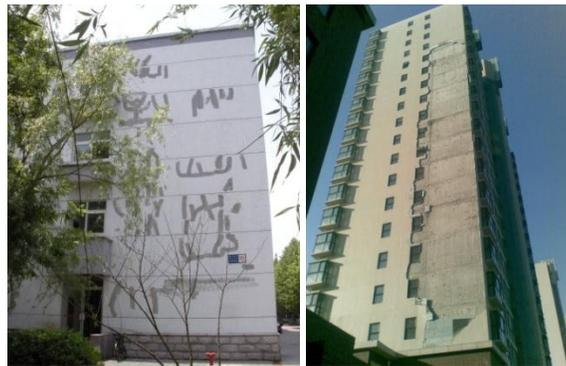
Fig.1 Damage of the covering plaster layer
