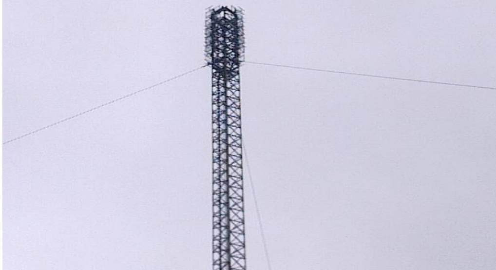
Figure.1 Nigeria Television Authority (NTA) Transmitting Antenna Ogbomosh.
