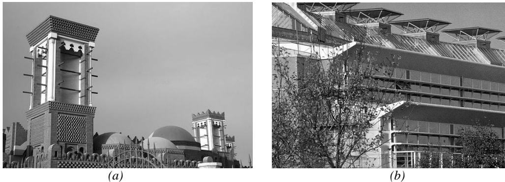
Figure 5: Applications of wind tower in; (a) vernacular architecture in Iran [30] (b) IONICA Building, UK [31]
