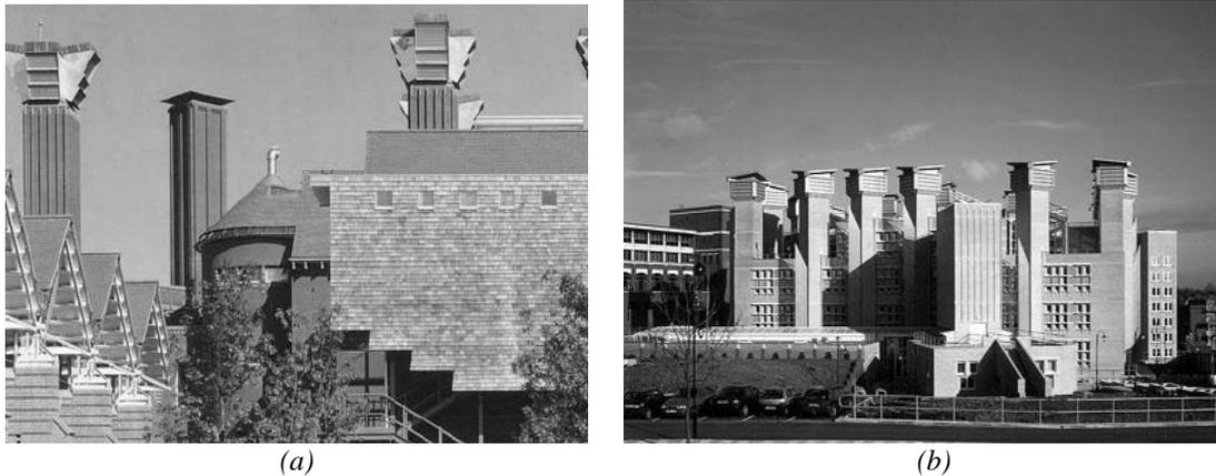
Figure 3: Actual application of stack ventilation towers at (a) The De Montfort University, UK [17] (b) Frederick Lanchester Library, UK [18]
